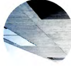
4 BOARD FORM CONCRETE
