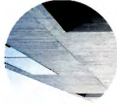
4 BOARD FORM CONCRETE
