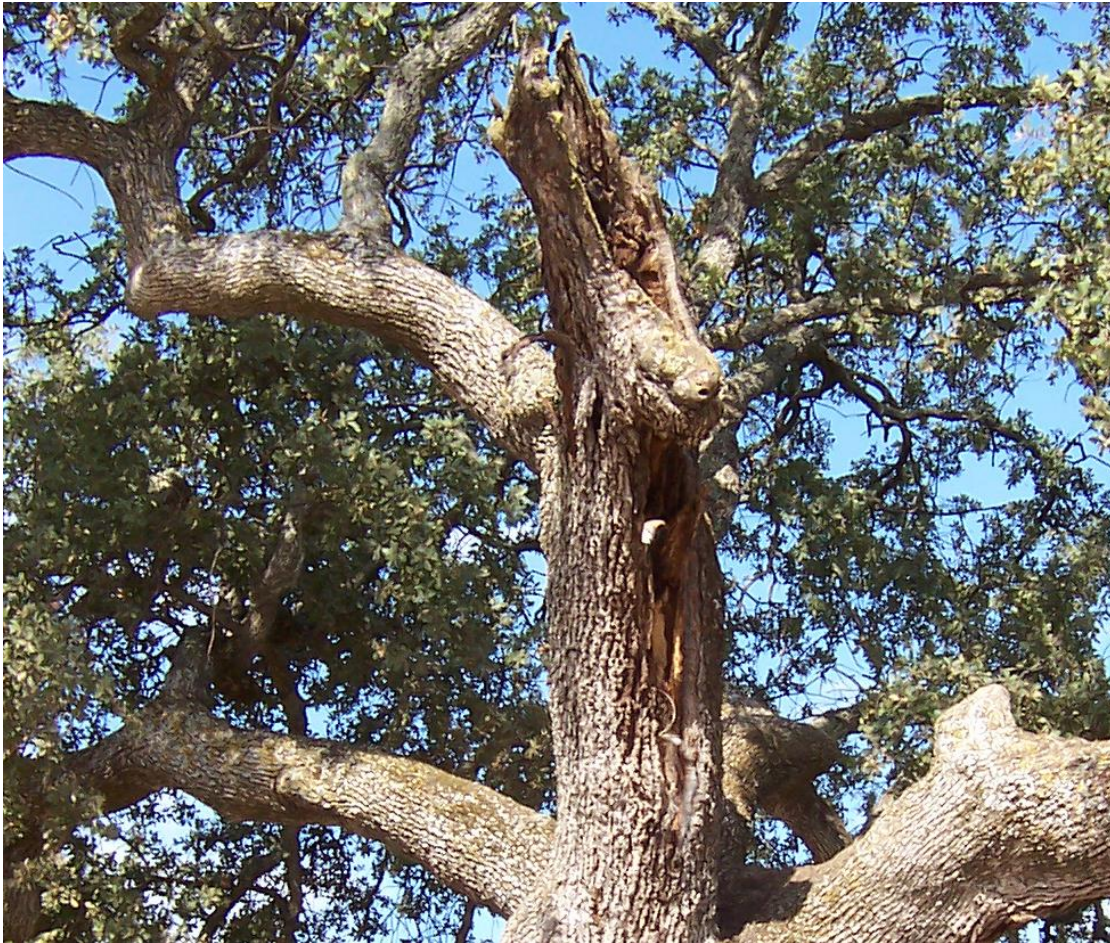
Priority 1 removals have defects such as extensive internal decay that cannot be cost-effectively or practically treated.
