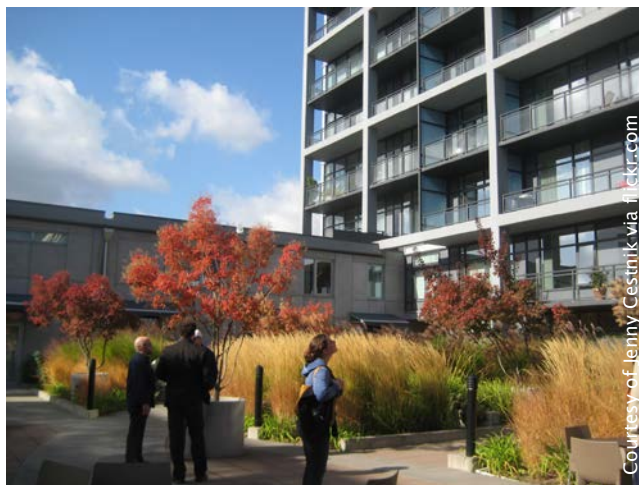
Exhibit 16. The Louisa, Portland, Oregon. This LEED Gold-certified, mixed-use building in Portland's Pearl District has a green roof that serves as a private outdoor gathering place for residents while reducing stormwater runoff and helping to cool the city.
