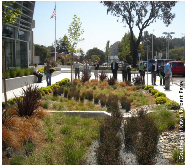
Exhibit 20. Brisbane City Hall, San Mateo County, California. Redesigning the parking lot for the Brisbane City Hall created space for a rain garden that captures stormwater from the building and parking lot. The redesigned parking lot accommodates the same number of cars. The city also gained an outdoor gathering space, room for bicycle parking, and a safer and more inviting entrance to the building.
