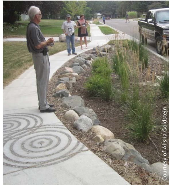
Exhibit 9. Green Street, Maplewood, Minnesota. Rain gardens along the curb capture stormwater from the street and make the neighborhood a more enjoyable place to walk.
