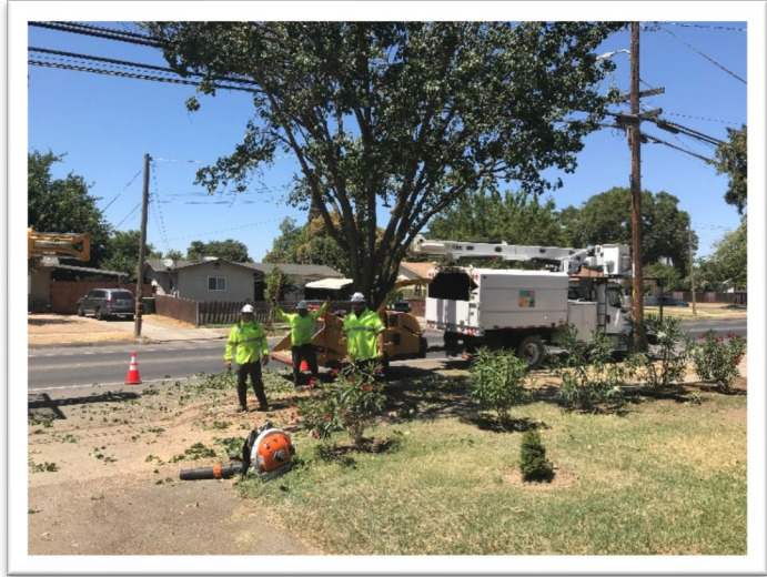
Tree trimming on Childs Avenue between Canal and N Streets
