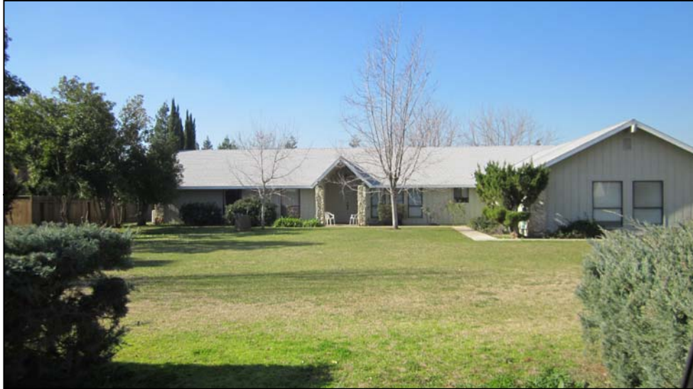
FIGURE 3.1-6 Residence in Remainder Area along Hatch Road
