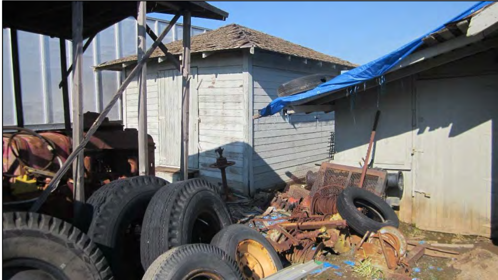
Outbuilding 4 South Elevation
