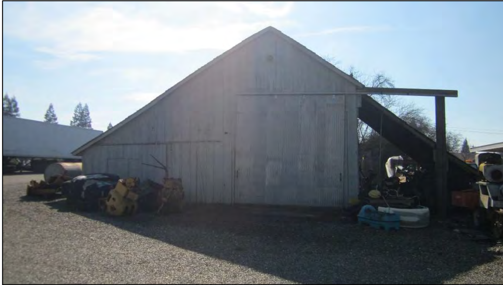
Outbuilding 3 North Elevation
