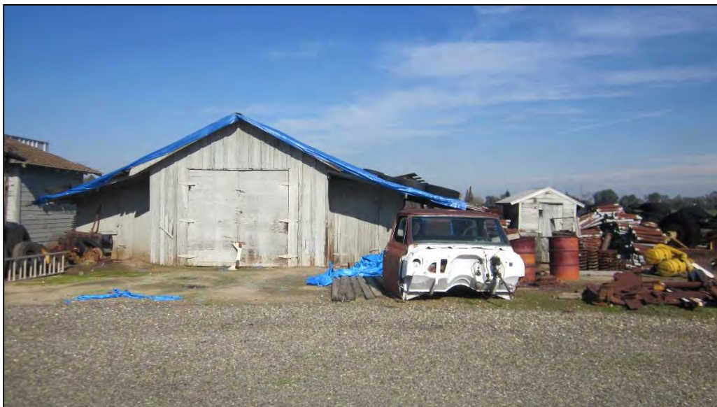
Outbuilding 5 South Elevation
