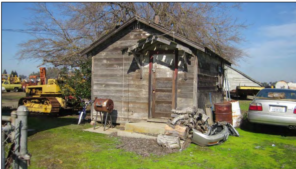
Outbuilding 1 South Elevation
