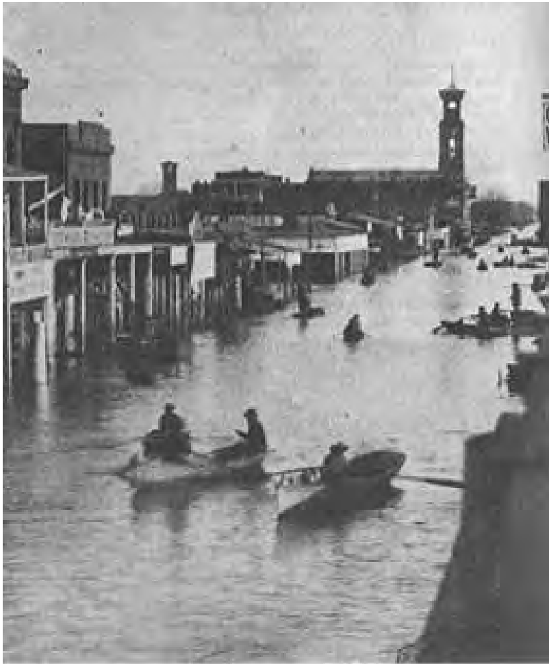
California flood of 1861-61, K Street, Sacramento. (USGS)
