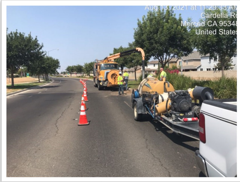
Park crews preforming irrigation repairs at Cardella Avenue median.
