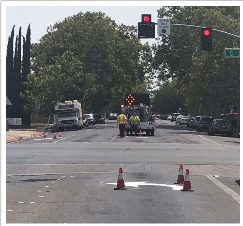
Street crews painting street legends/markings in various locations
