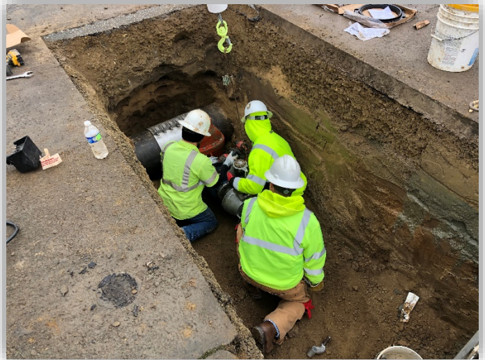
Crews tapped for a new water main crossing G Street just north of Yosemite Ave.
