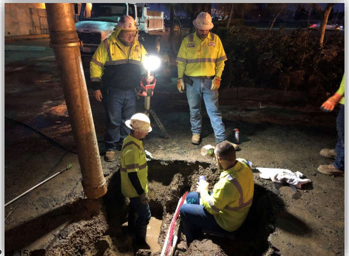
Crews repaired an irrigation leak behind Five Guys Restaurant
