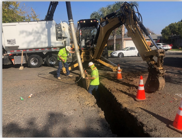
Crews replaced a leaking 1” copper service line at Partridge Dr.
