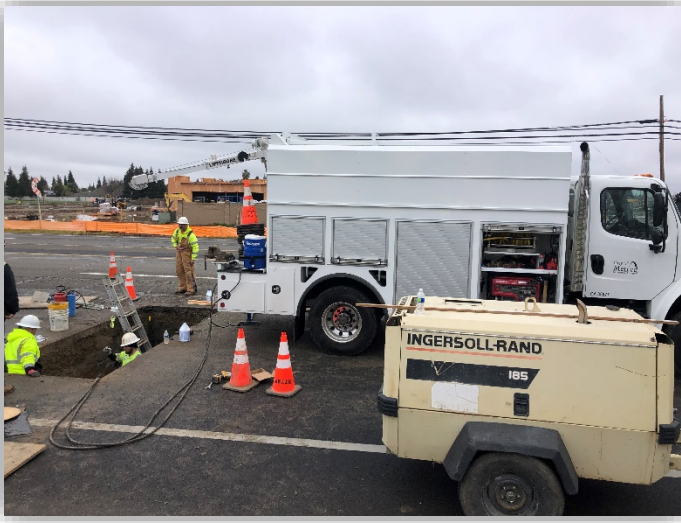
Crews tapped for a new water main crossing G Street just north of Yosemite Ave.
