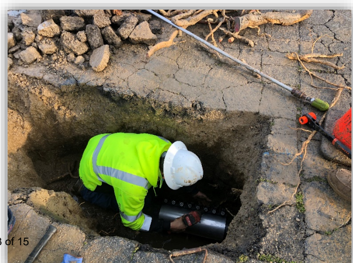
Crews repaired a service leak near 8 th and S Streets.
