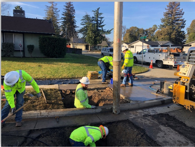
Crews repaired a service leak near 8 th and S Streets.
