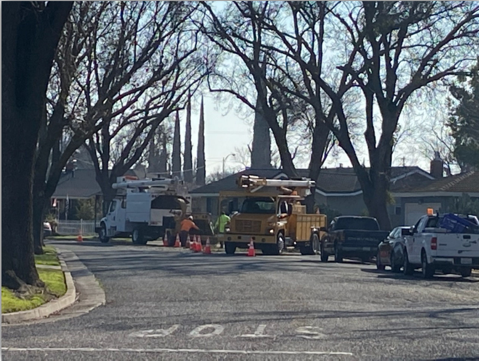
Tree Crews working in the Brookdale Avenue area.
