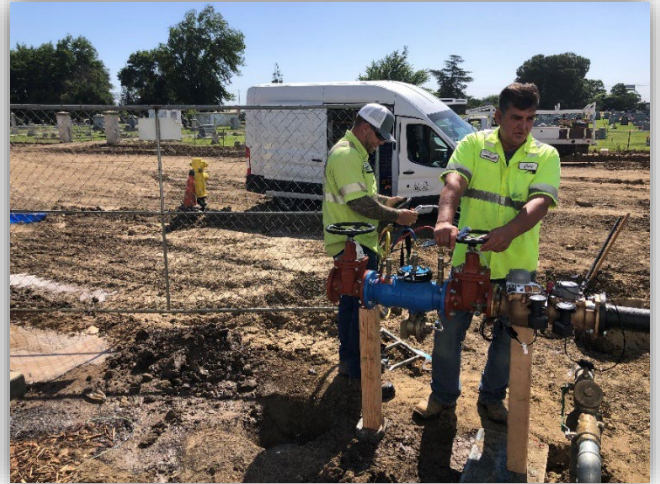
Backflow Testing
