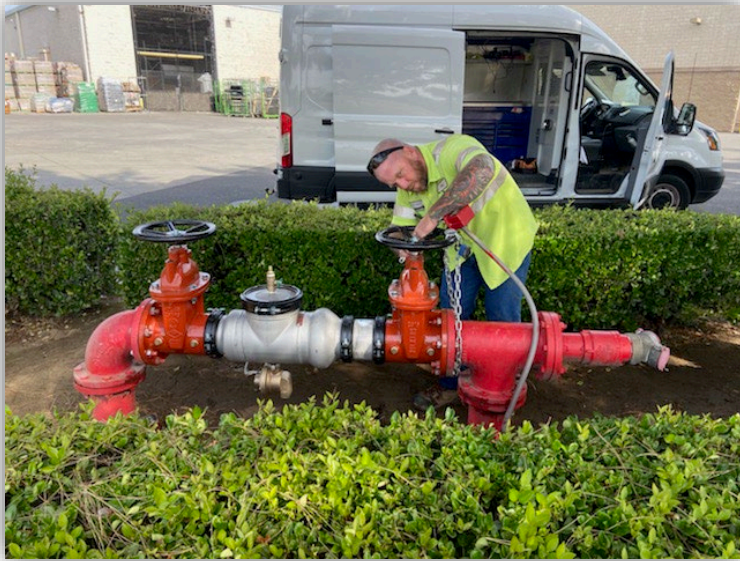
Water backflow crew replaced a failing 6" Fire Service.
