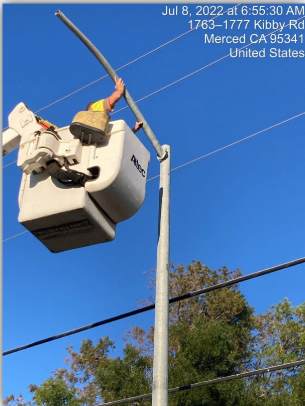
Street Crews replaced a streetlight pole on Kibby Ave.
