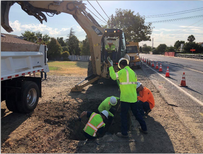
Crews upgraded water service line from 1" to 2" on Nashville Court
