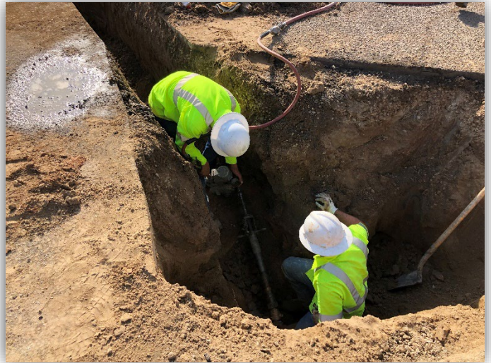
Crews tapped and installed a water service line on S. Coffee Street
