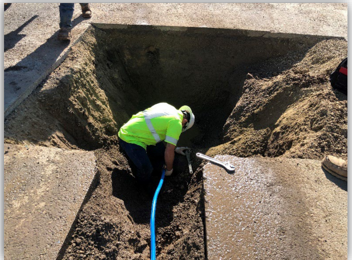
Crews tapped and installed a water service line on S. Coffee Street
