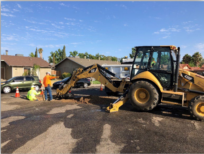
Crews tapped and installed a water service line on S. Coffee Street
