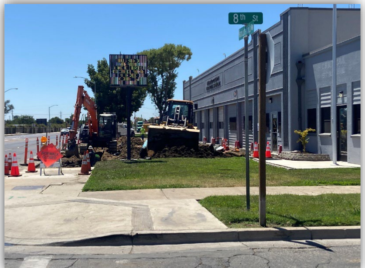
More photos of the replacement of a water main section along Martin Luther King, Jr. Way in front of the Merced County Fire Station.
