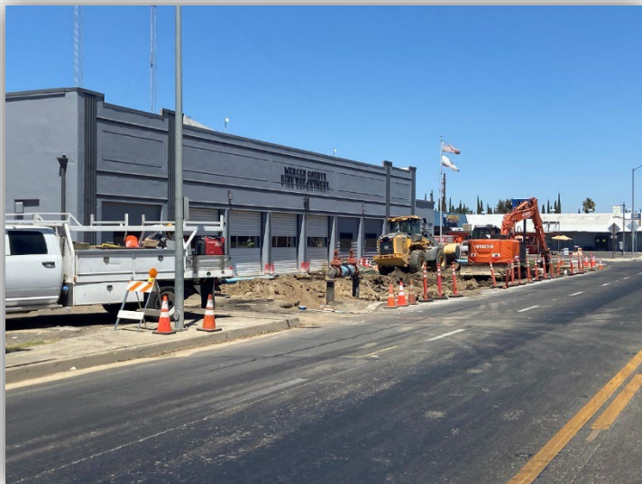
More photos of the replacement of a water main section along Martin Luther King, Jr. Way in front of the Merced County Fire Station.
