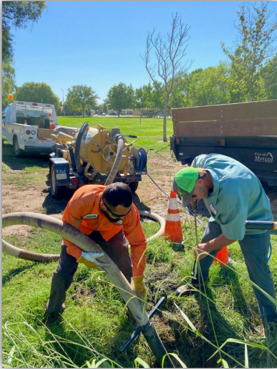
Park Crews repaired a main line at Rahilly Park.
