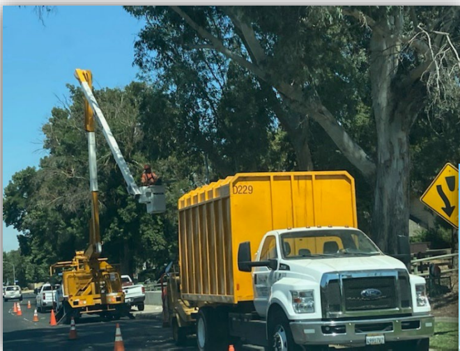
Crews pruned the Eucalyptus Grove along M Street
