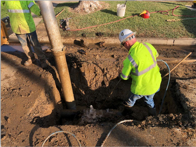
Crews repaired a 6” water main line at the 2500 block of I Street
