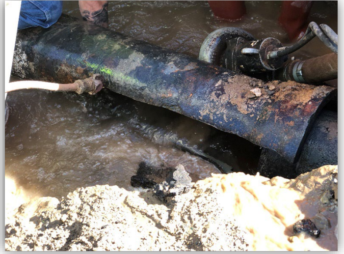
Crews repaired a 10” water main line at the 500 block of W. Childs Ave
