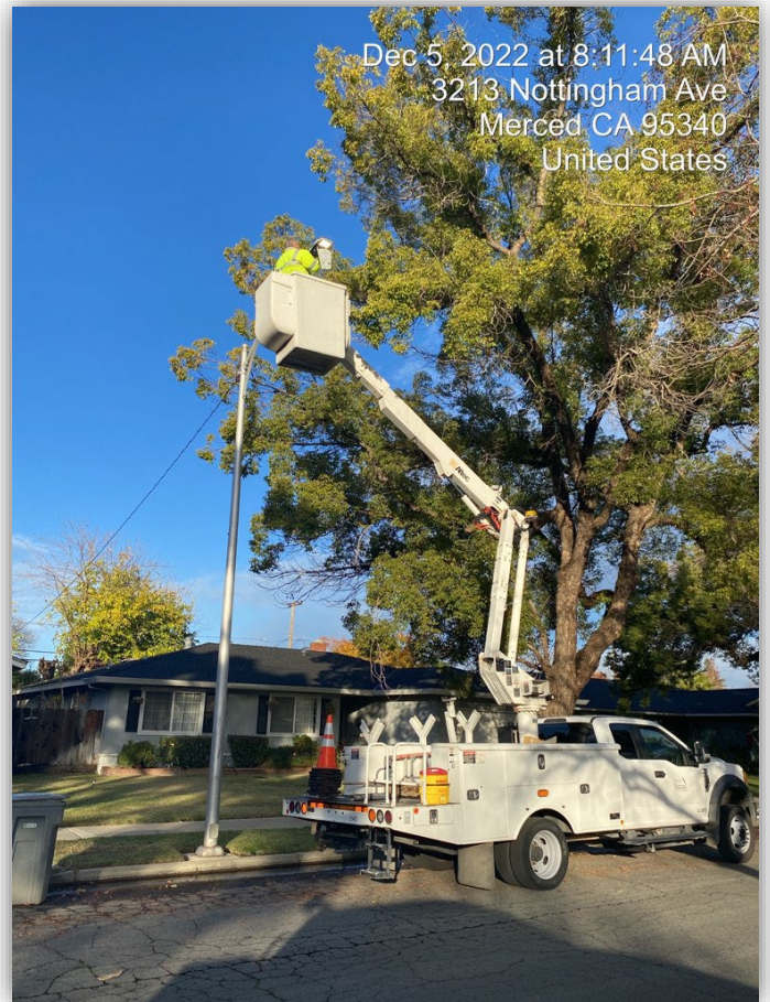
Street Crews repaired a streetlight on Nottingham Ave.
