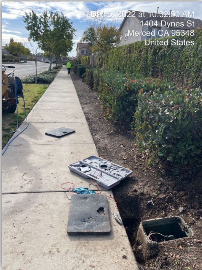
Parks Crews repaired irrigation wiring along St. Augustine
