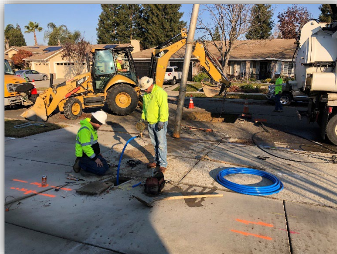
A 1” water service line was replaced at Redwing Dr.
