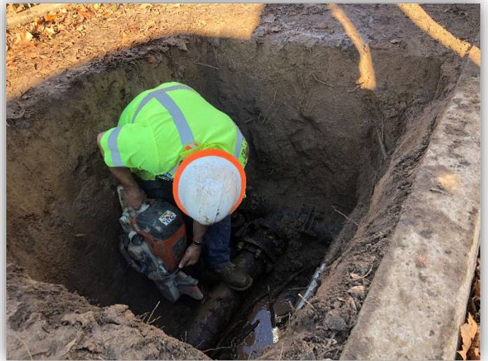
A damaged fire hydrant was replaced at McKee Rd.
