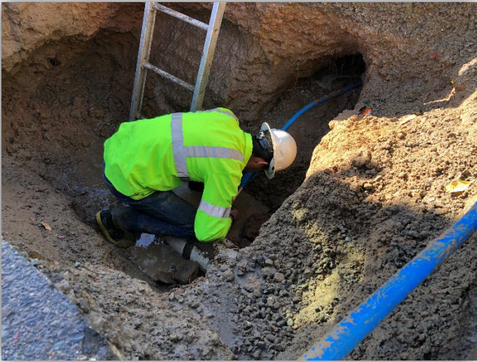
Water crews replaced a 1” water service line at Santa Nella Ct.
