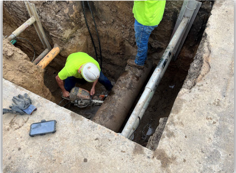
Crews tapped into a 16” water main line for a new 10” water Service at Mission Rd and Tyler Ave.
