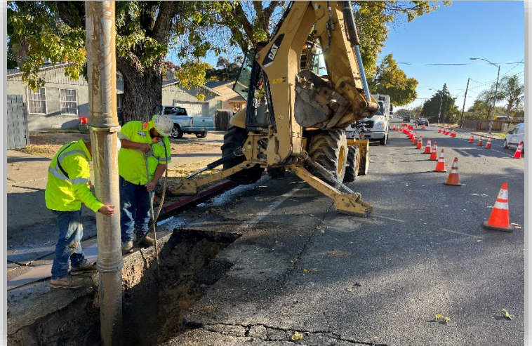
Crews repaired a 10” water main line break at the 1000 block of W. Childs Ave.
