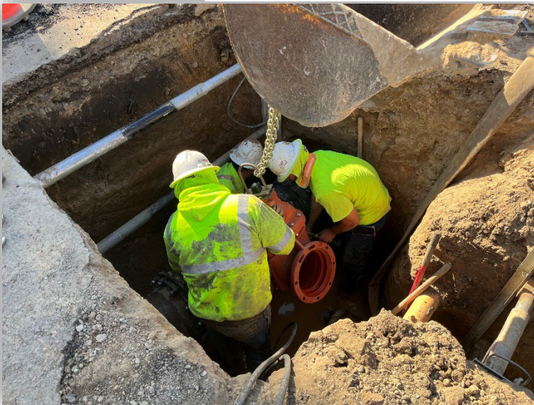
Crews tapped into a 16” water main line for a new 10” water Service at Mission Rd and Tyler Ave.
