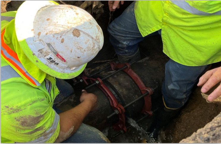
Crews repaired a 10” water main line break at the 1000 block of W. Childs Ave.
