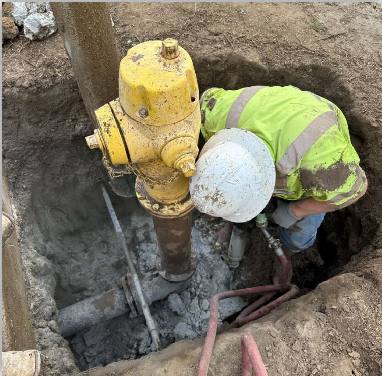
Crews replaced a defective fire hydrant at W. North Bear Creek and Hwy 99.
