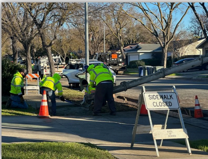
Street crews repaired a section of sidewalk on Kernland Ave
