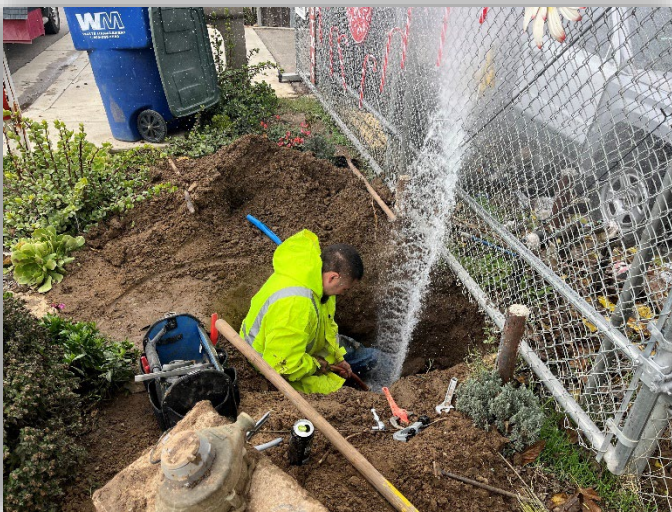
A 1" water service line was repaired on the 3800 block of Hwy 140.
