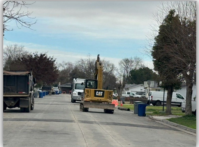
Water crews worked on Bel Air Drive
