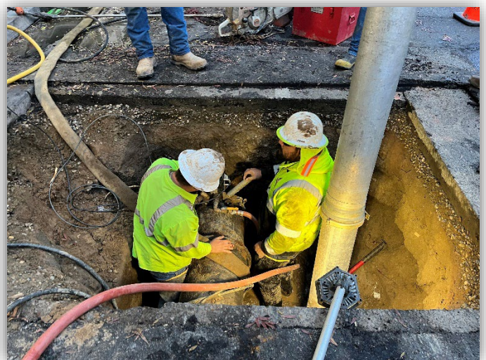
Water crews worked in conjunction with a contractor to relocate a water main and install new fire hydrants on Bel Air Drive
