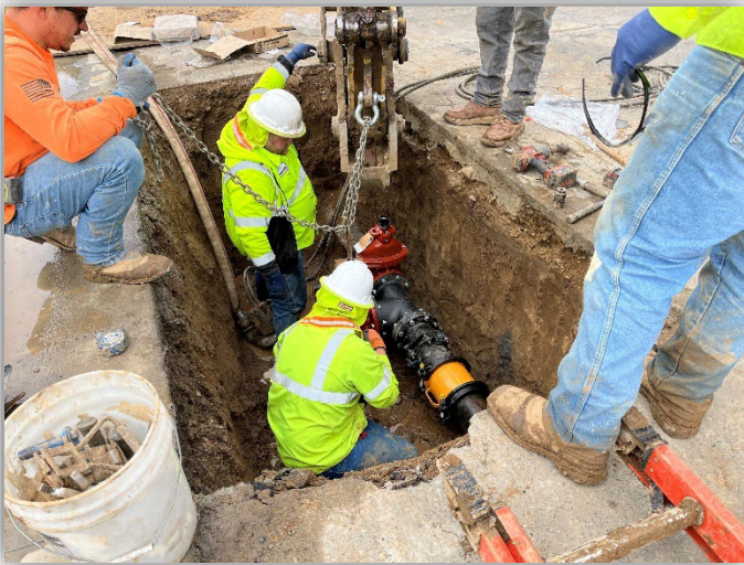
Water crews worked in conjunction with a contractor to relocate a water main and install new fire hydrants on Bel Air Drive
