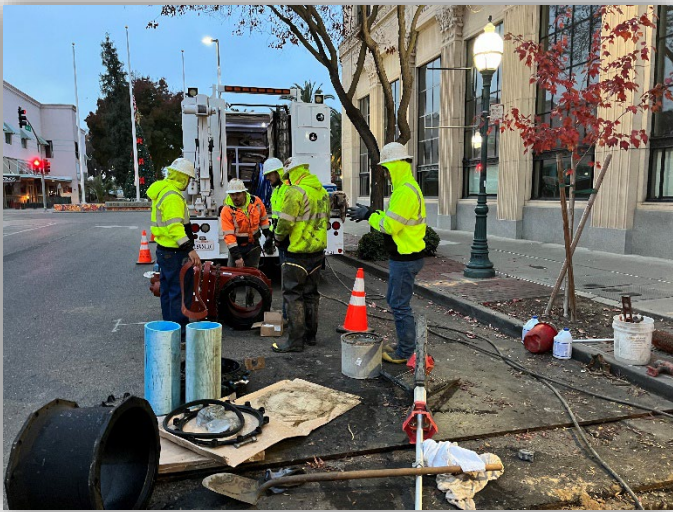
New 16” water main valve was installed near Canal and Main Streets.
