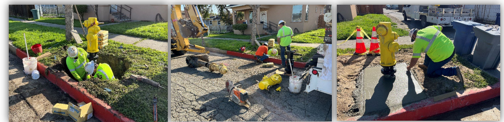
Water department flushed water main lines in the southeast area of Merced
