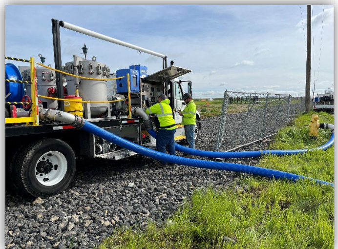
Water department flushed water main lines in the southeast area of Merced
