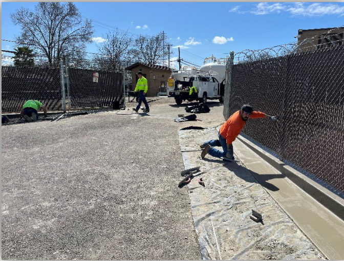
Water department performed improvements at Wellsite 3
