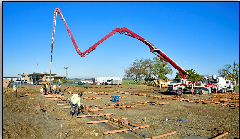
This week marked a significant milestone in constructing the replacement terminal at Merced Yosemite Regional Airport with the installation of concrete footings and pedestals.
