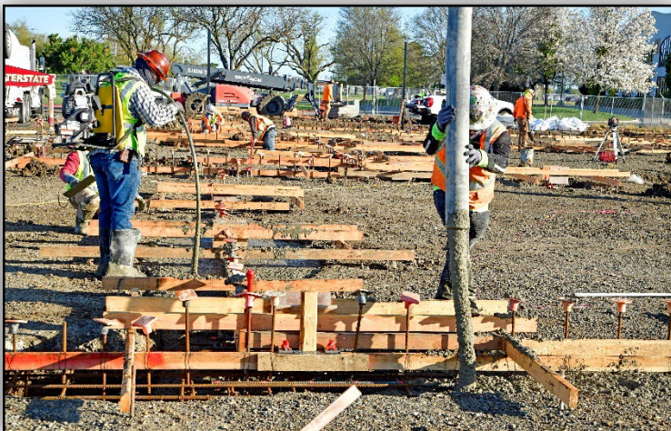
This week marked a significant milestone in constructing the replacement terminal at Merced Yosemite Regional Airport with the installation of concrete footings and pedestals.
