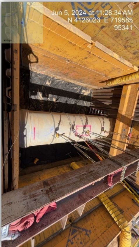
Crew installing a 10-foot diameter manhole at the Wastewater Treatment Plant
