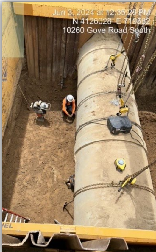
Crew installing a 10-foot diameter manhole at the Wastewater Treatment Plant
