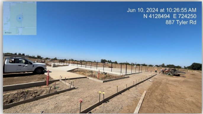
Community Park 42- Crew working on Futsal Court, finishing up the curb and gutter in the parking area, installing waterlines and grading.
