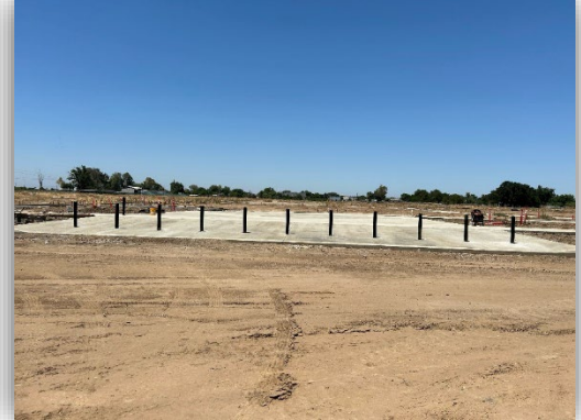
Merced Yosemite Regional Airport- Crews installed metal beams for the outer walls.
