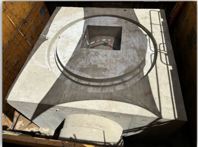
Wastewater Treatment Plant- Crews removed the forms from the manhole foundation and prepared for coating.
