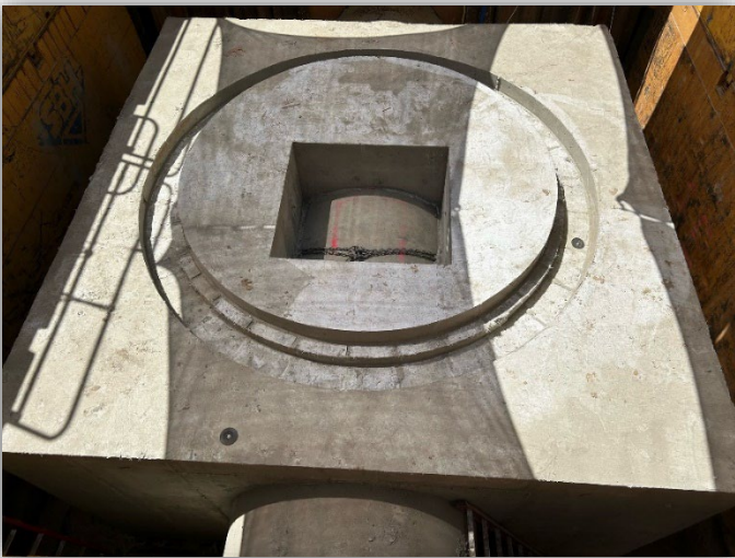
Wastewater Treatment Plant- Crews removed the forms from the manhole foundation and prepared for coating.
