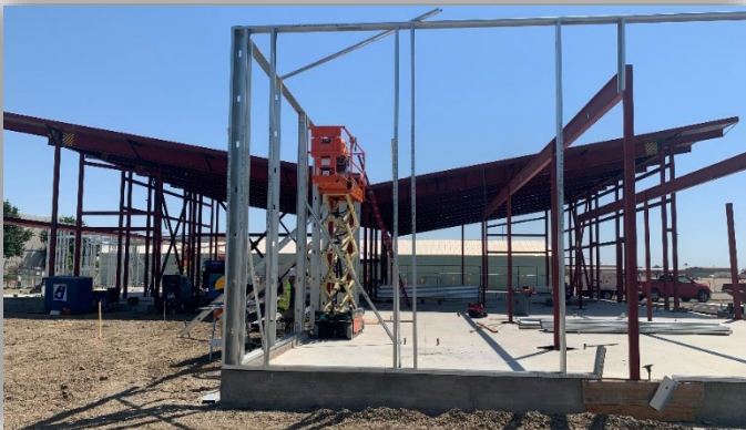
Merced Yosemite Regional Airport- Crews installed metal beams for the outer walls.
