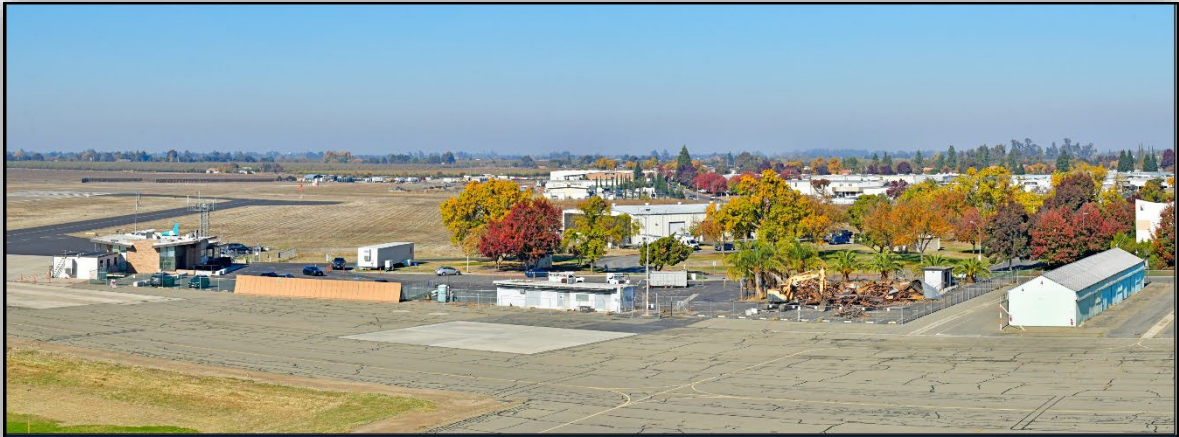
Continued progress at Merced Yosemite Regional Airport Terminal Replacement Project.
