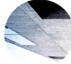
4 BOARD FORM CONCRETE
