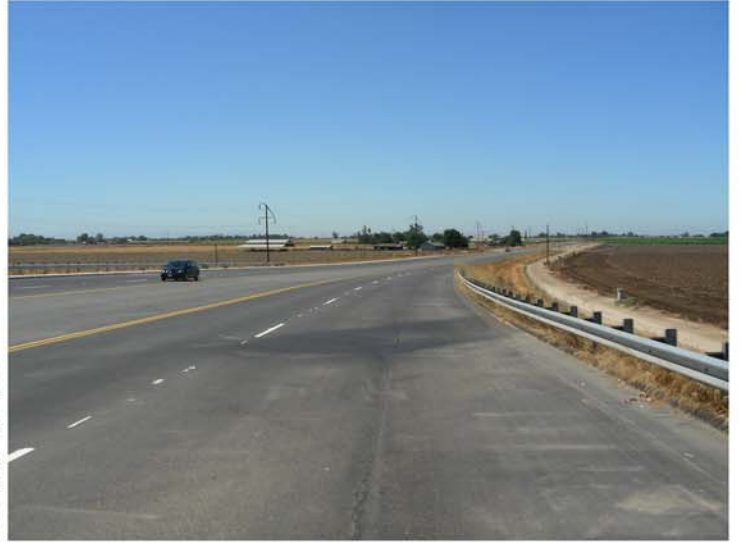
Highway 99 and Mission Ave Looking West (P #19)
