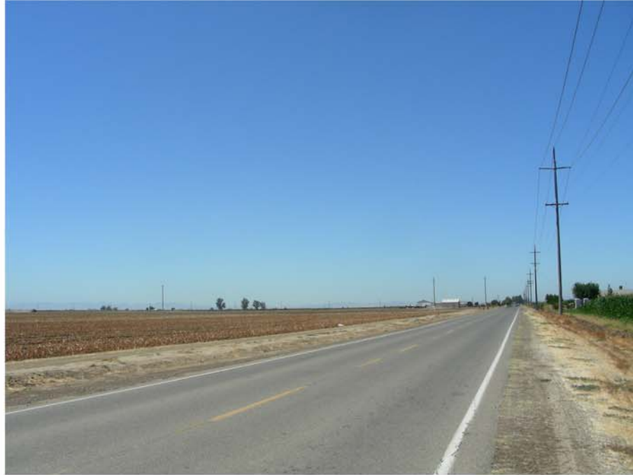
Dickenson Ferry Road South of Merced Regional Airport Looking West (P #16)
