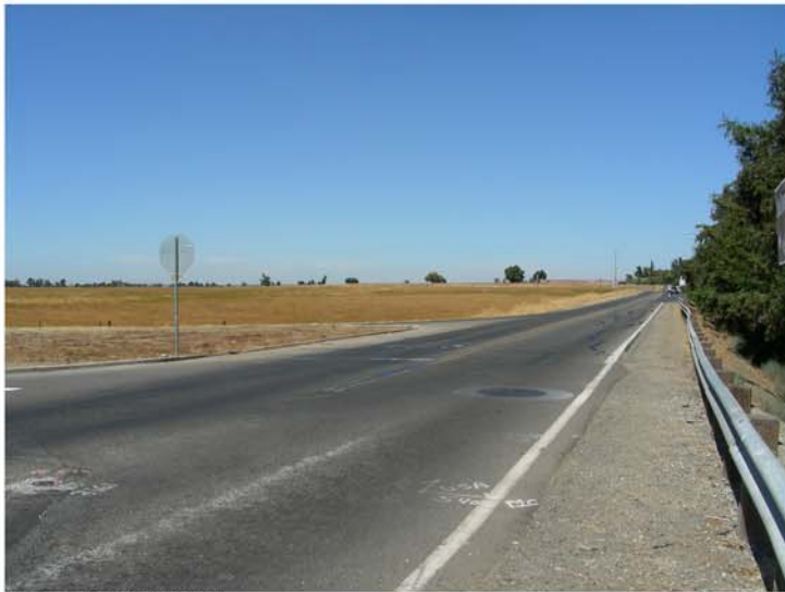
Bellevue Road and North Lake Road Looking North (P #3)
