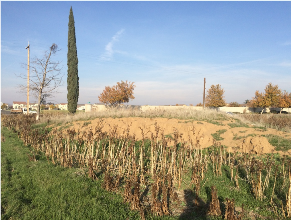
Photograph 11: View of debris, trees, and electrical pole associated with demolished structure; facing north
