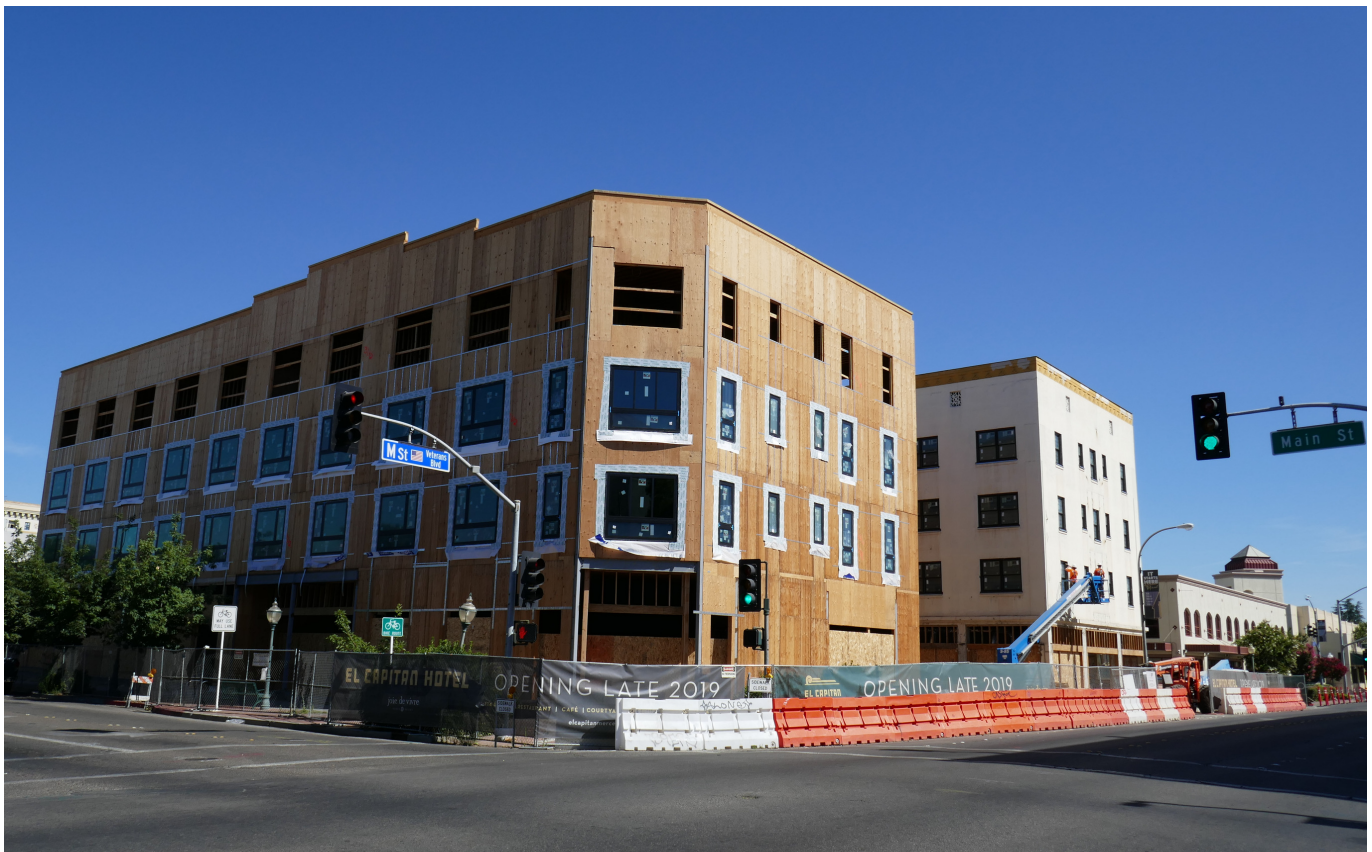
El Capitan Hotel Under Construction - Downtown Merced
