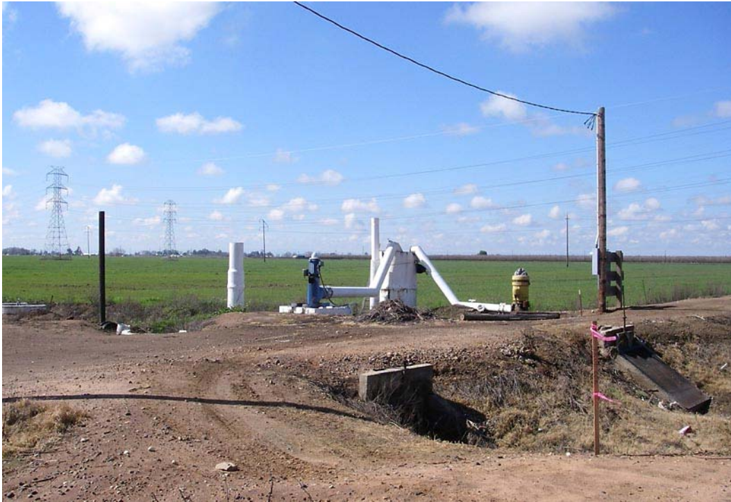
View Point 4 - Southwest View from Childs/Tower - Existing
