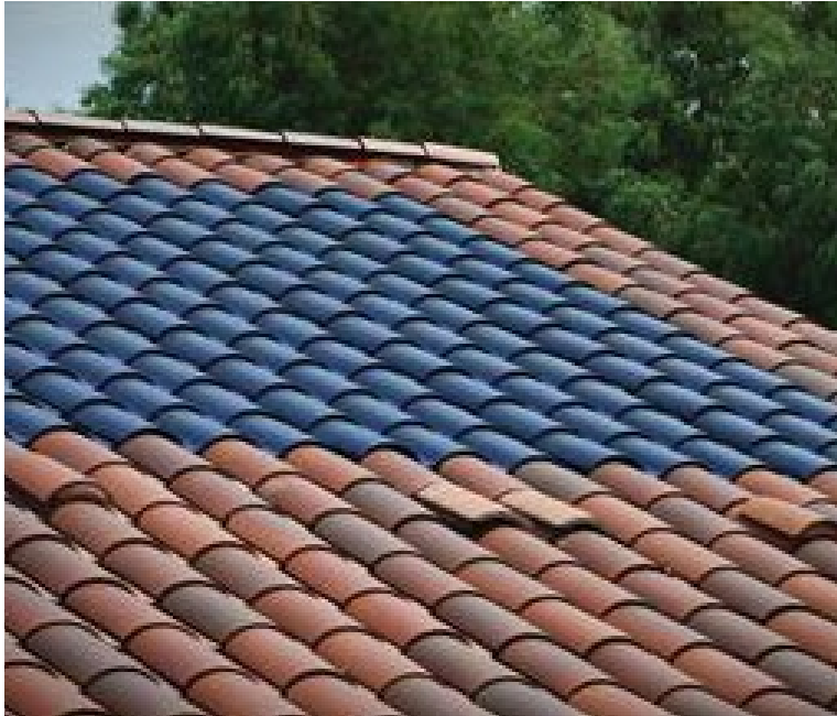
Solar panels integrated into roof tiles
