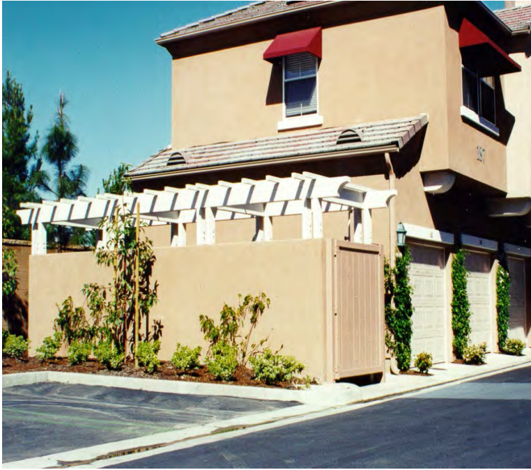
Screening is consistent with the surrounding architecture
