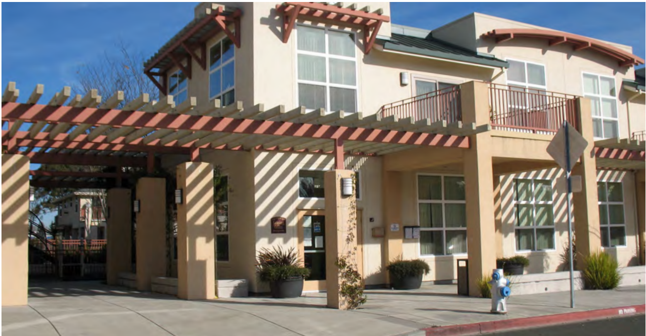
Building fronts the sidewalk and provides
