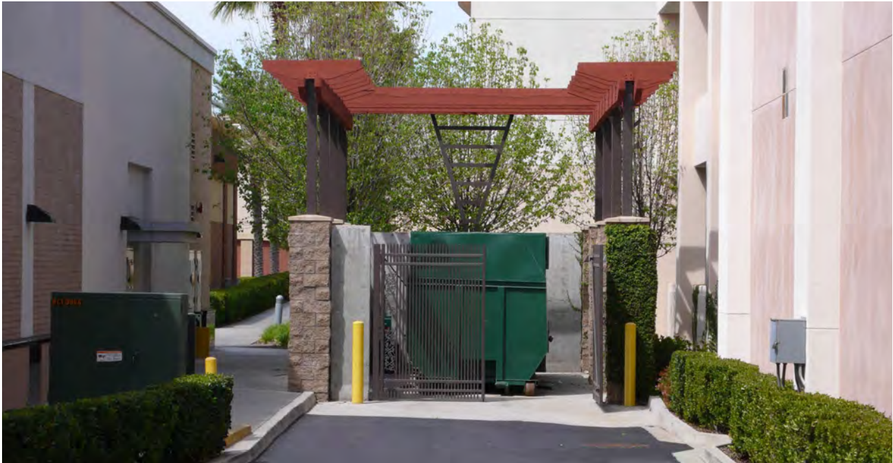
Enclosure is located to the side of the primary building, with a clear path for mechanical pickup
