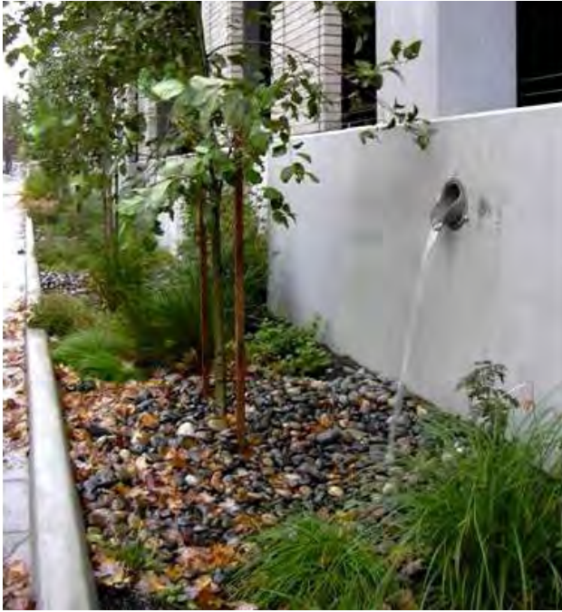
Roof downspout empties into planter
