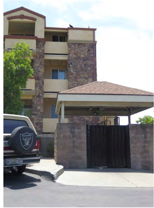
Waste enclosure is within 150 feet of units
