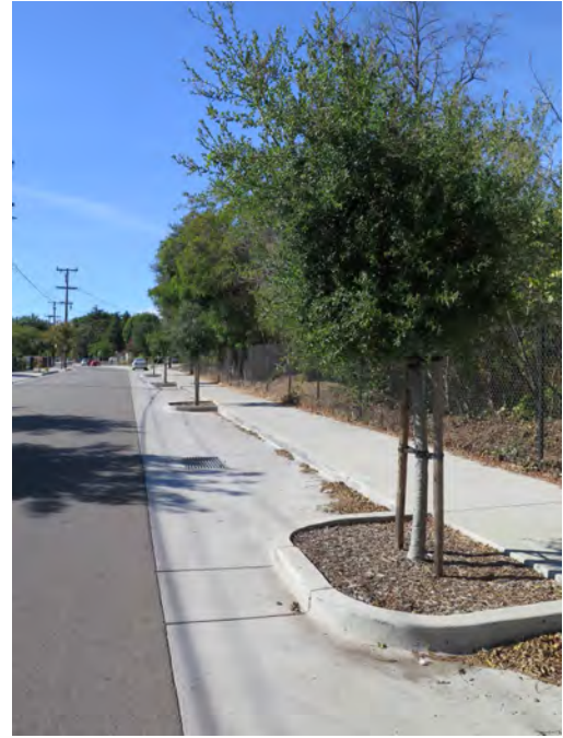
Curbed tree wells between parking spaces
