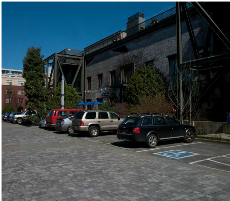
Permeable paving in parking area
