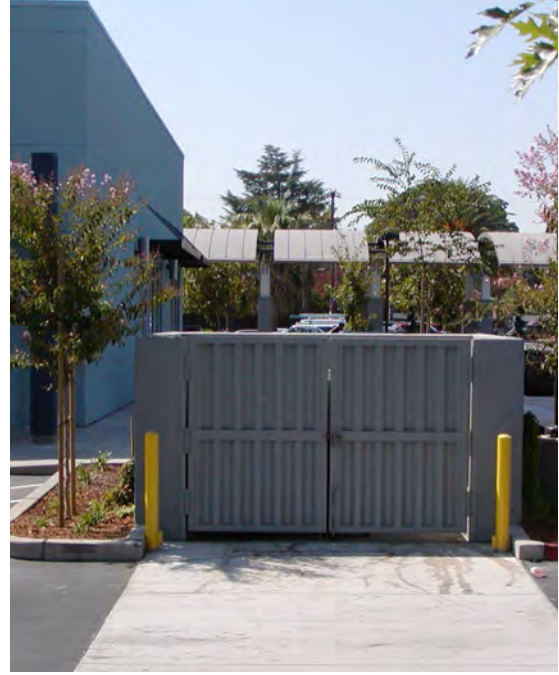
Curb and metal bollards to protect enclosure
