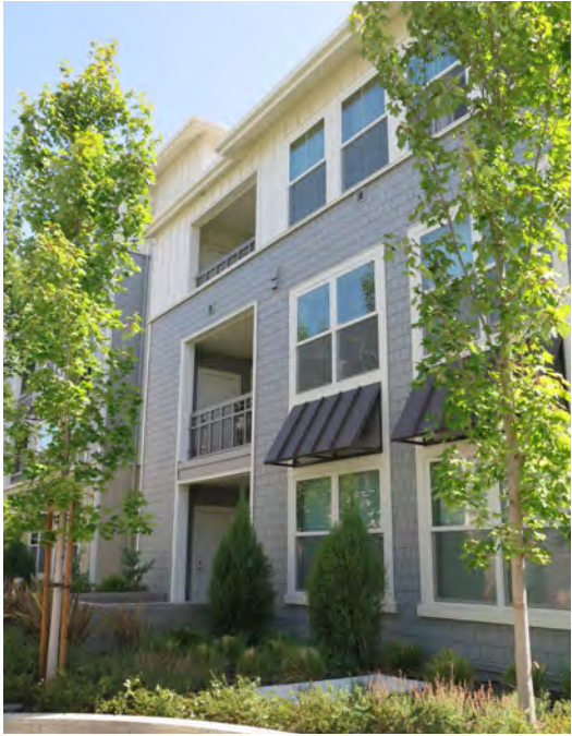
Narrow canopy trees along multi-story building
