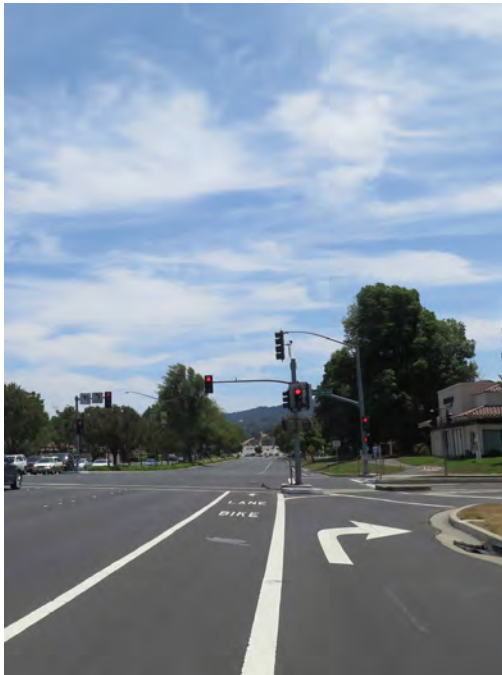
Bike lane positioned left of right-turn lane
