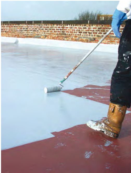
Applying liquid cool roof coating
