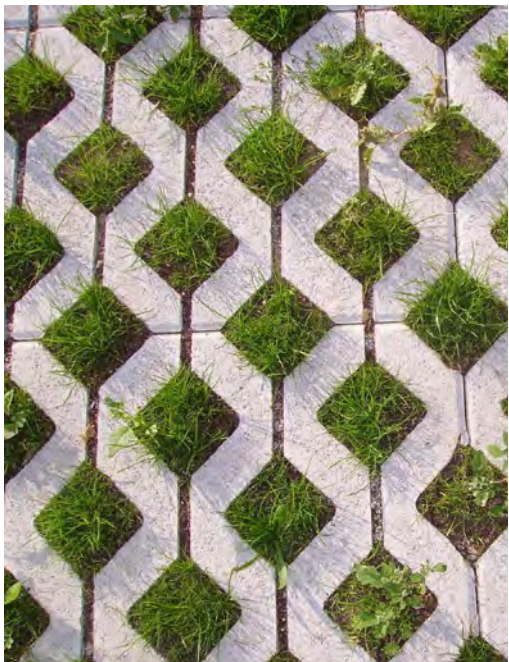
Turf block pavers used in parking area
