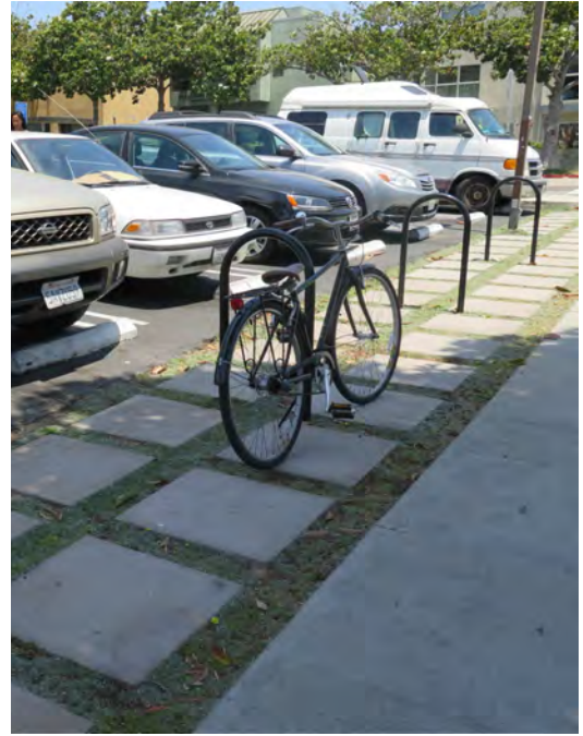
Inverted U-shaped bicycle rack
