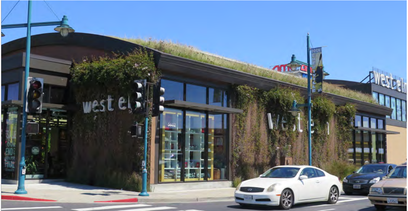
Vegetation on a sloped roof ensures proper drainage
