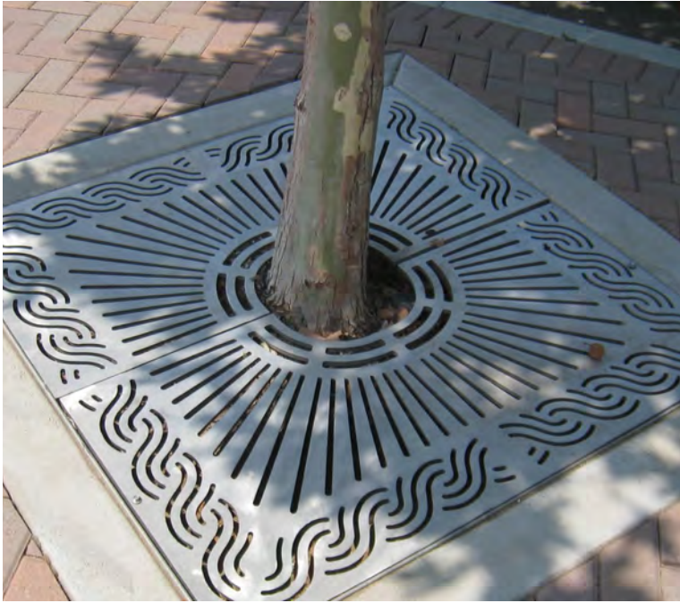
Tree grates used in commercial areas
