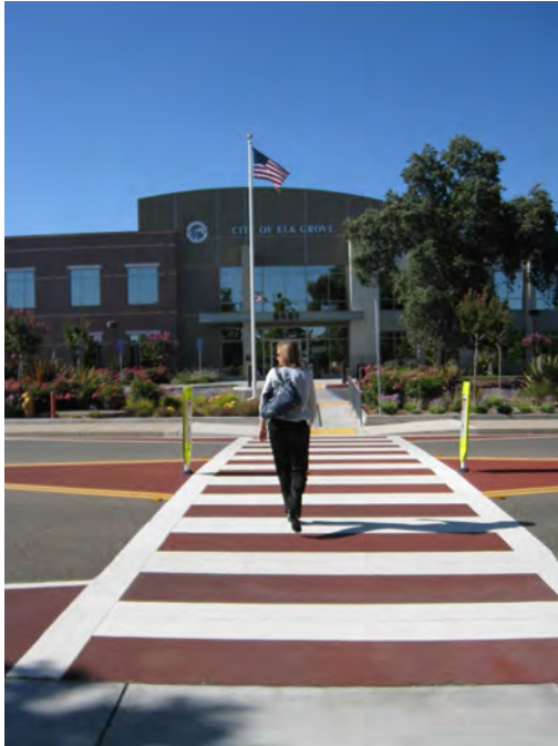
Bold painted striping delineates crosswalk
