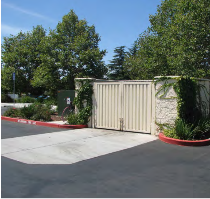
Concrete pad in front of enclosure
