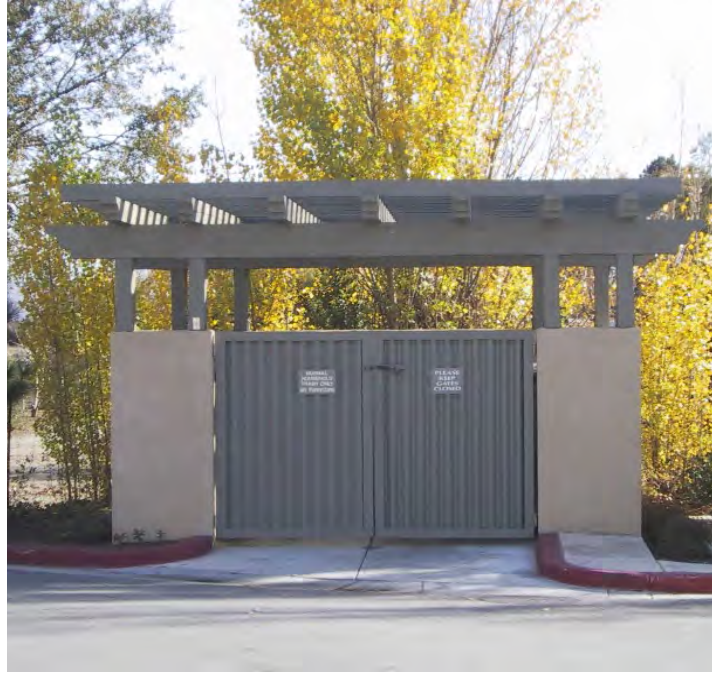
Trellis screens the enclosure from upper stories
