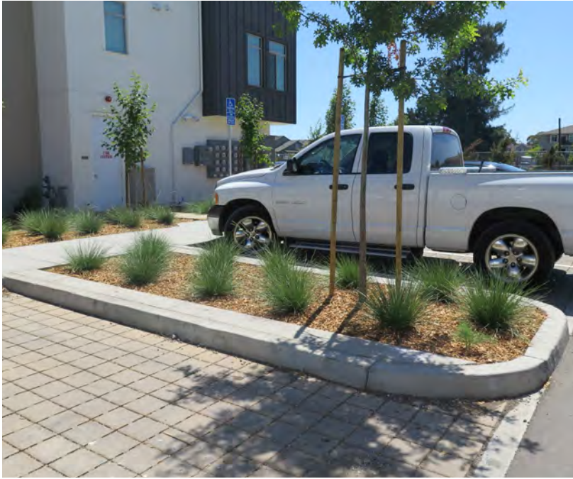
Permeable paving used in parking areas
