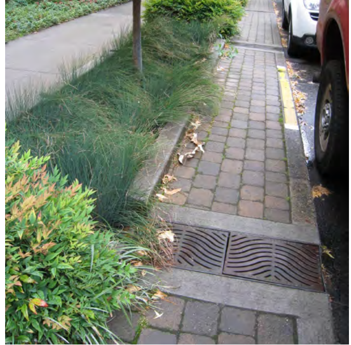
Stormwater planter between curb and sidewalk
