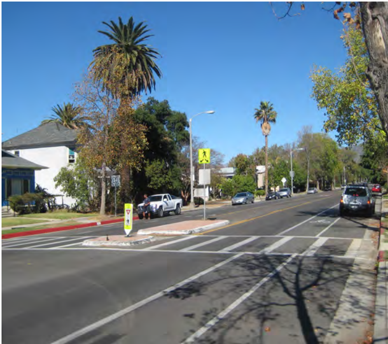
"Complete Street" featuring vehicle, bike, and pedestrians facilities
