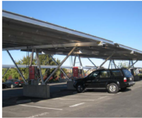
Solar panels serve as shade structures in parking lots
