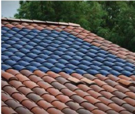
Solar panels integrated into roof tiles
