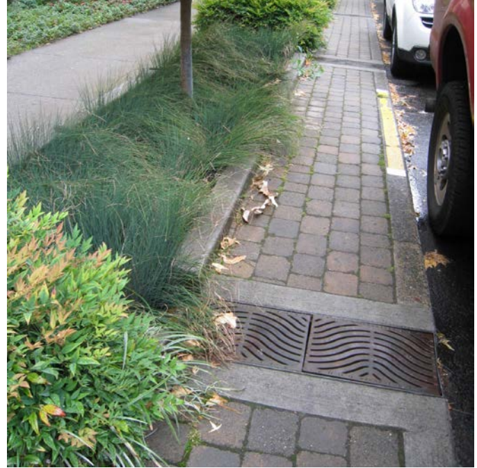
Stormwater planter between curb and sidewalk
