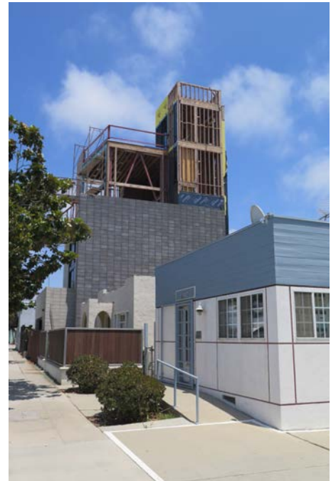
New development does not match scale of existing buildings
