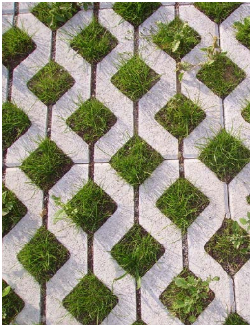
Turf block pavers used in parking area
