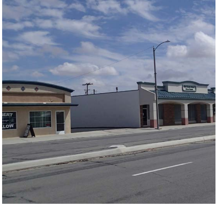
Shared driveway between adjoining sites
