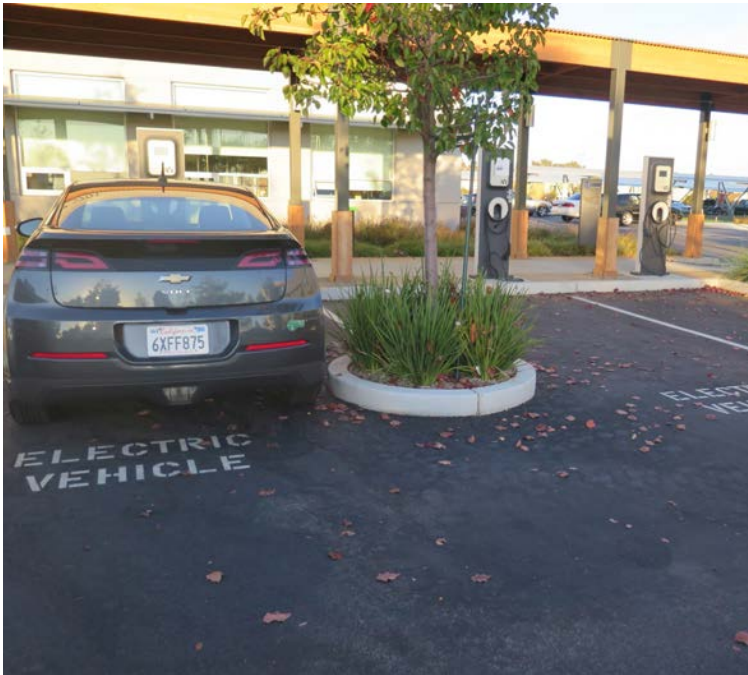
Designated parking for electric vehicles
