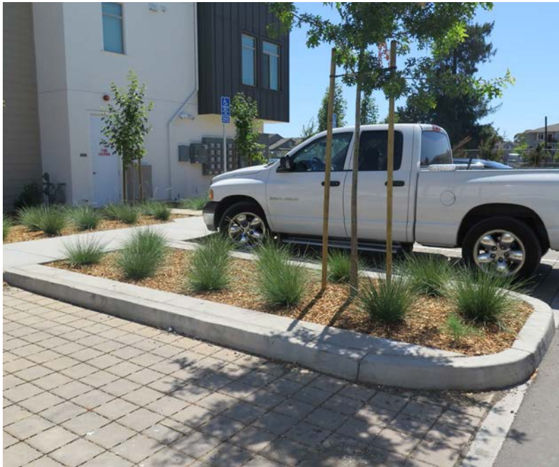
Permeable paving used in parking areas
