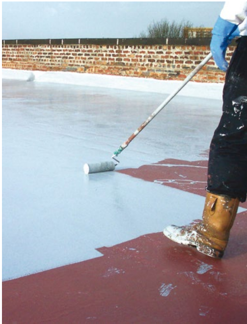
Applying liquid cool roof coating
