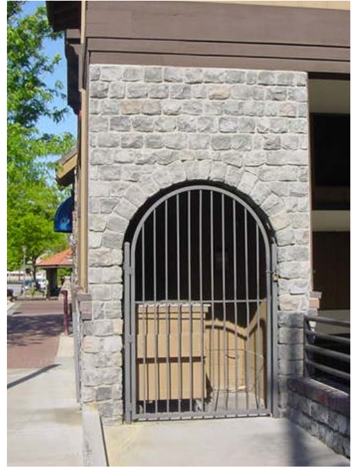
Decorative iron pedestrian gate
