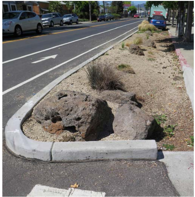
This bioswale does not provide enough vegetation
