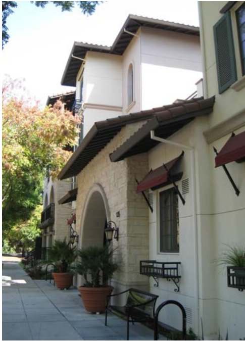
Awnings provide shelter
