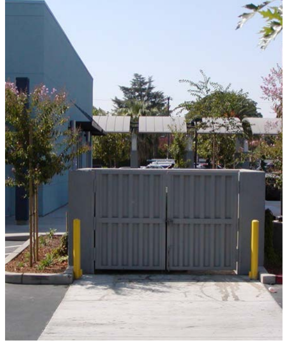
Curb and metal bollards to protect enclosure
