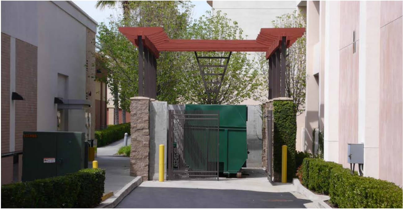
Enclosure is located to the side of the primary building, with a clear path for mechanical pickup
