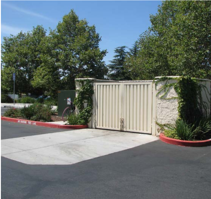
Concrete pad in front of enclosure
