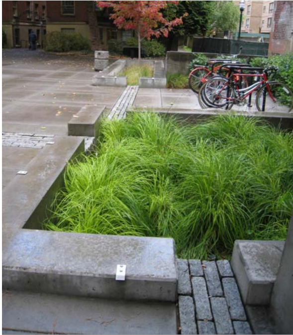
Stormwater planter with grasses
