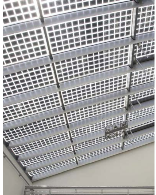
Solar panels integrated into glazing
