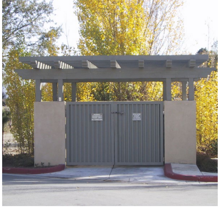
Trellis screens the enclosure from upper stories
