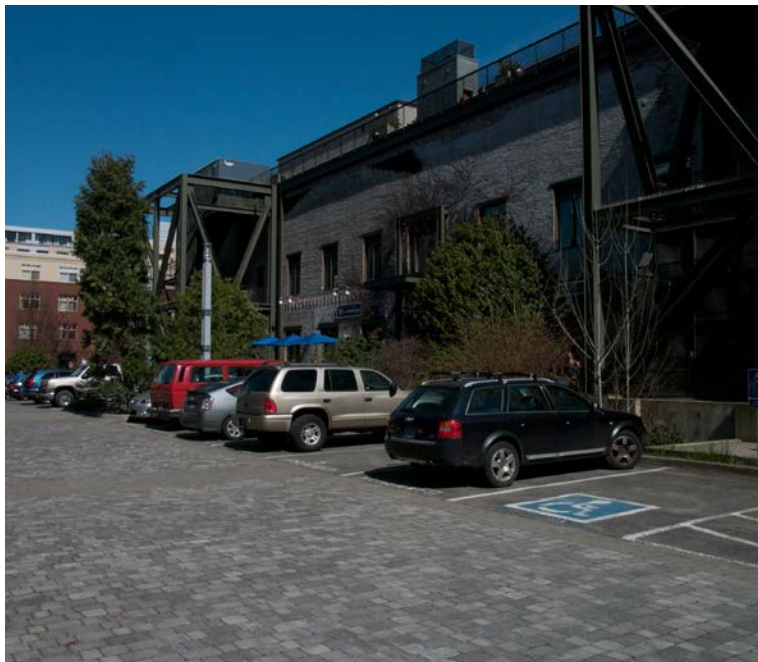
Permeable paving in parking area
