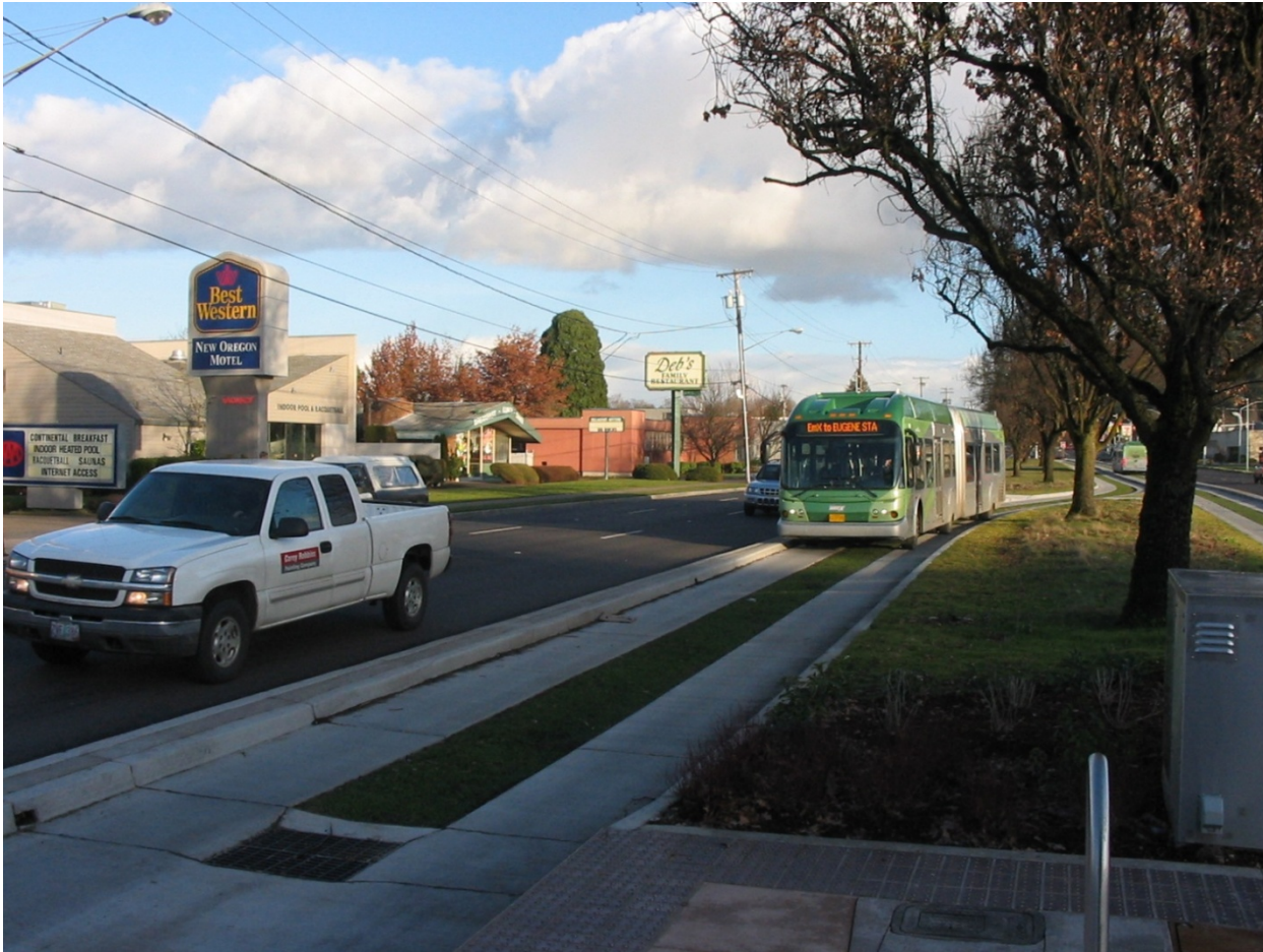
Figure 1-9 BRT Median Transitway Example: Eugene EMX
