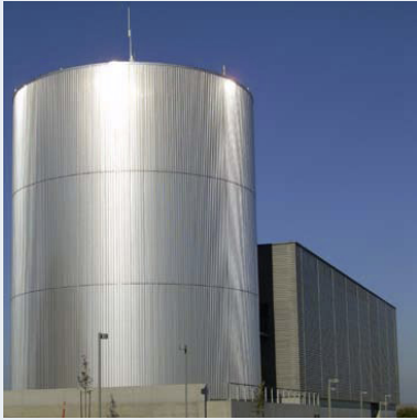
Image of UC Merced's Central Plant received a LEED Gold rating
