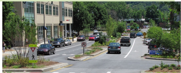
Curb extensions and median make crossing four-lane streets safer and more manageable. (Credit: Dan Burden)
