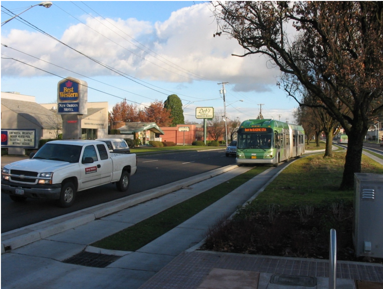
Figure 1-8 BRT Median Transitway Example: Eugene EMX
