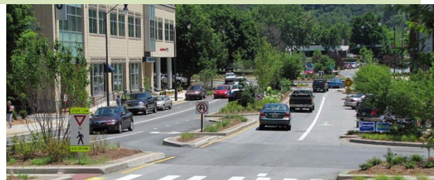
Curb extensions and median make crossing four-lane streets safer and more manageable.
