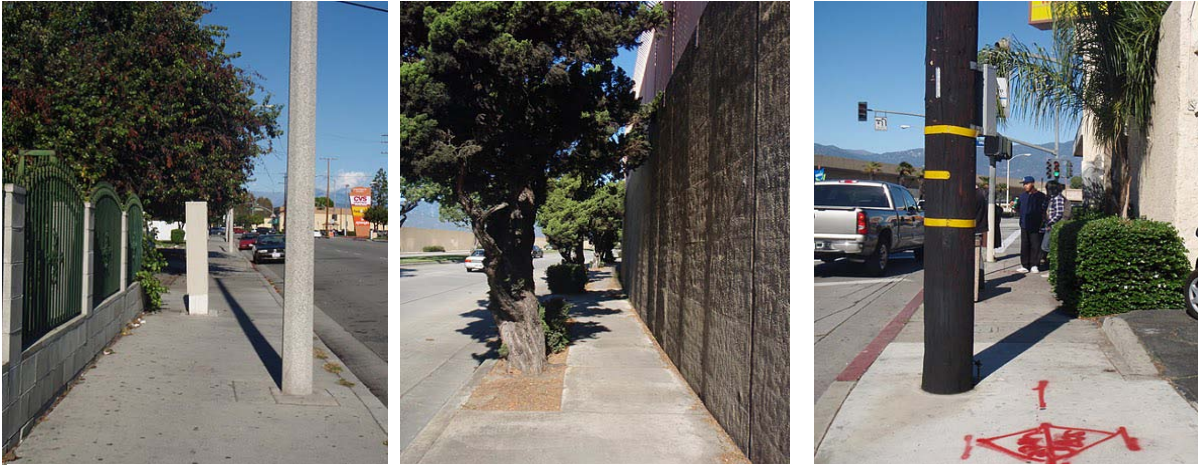
Sidewalks constructed without adequate design guidelines (Credit: Chanda Singh)
