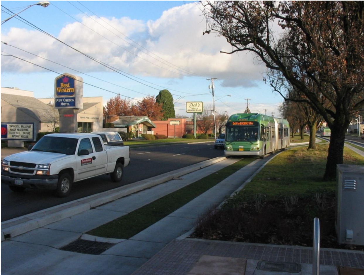
Figure 1-9 BRT Median Transitway Example: Eugene EMX
