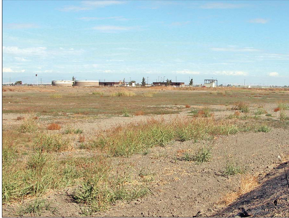
View of the WWTP facilities and surrounding lands.
