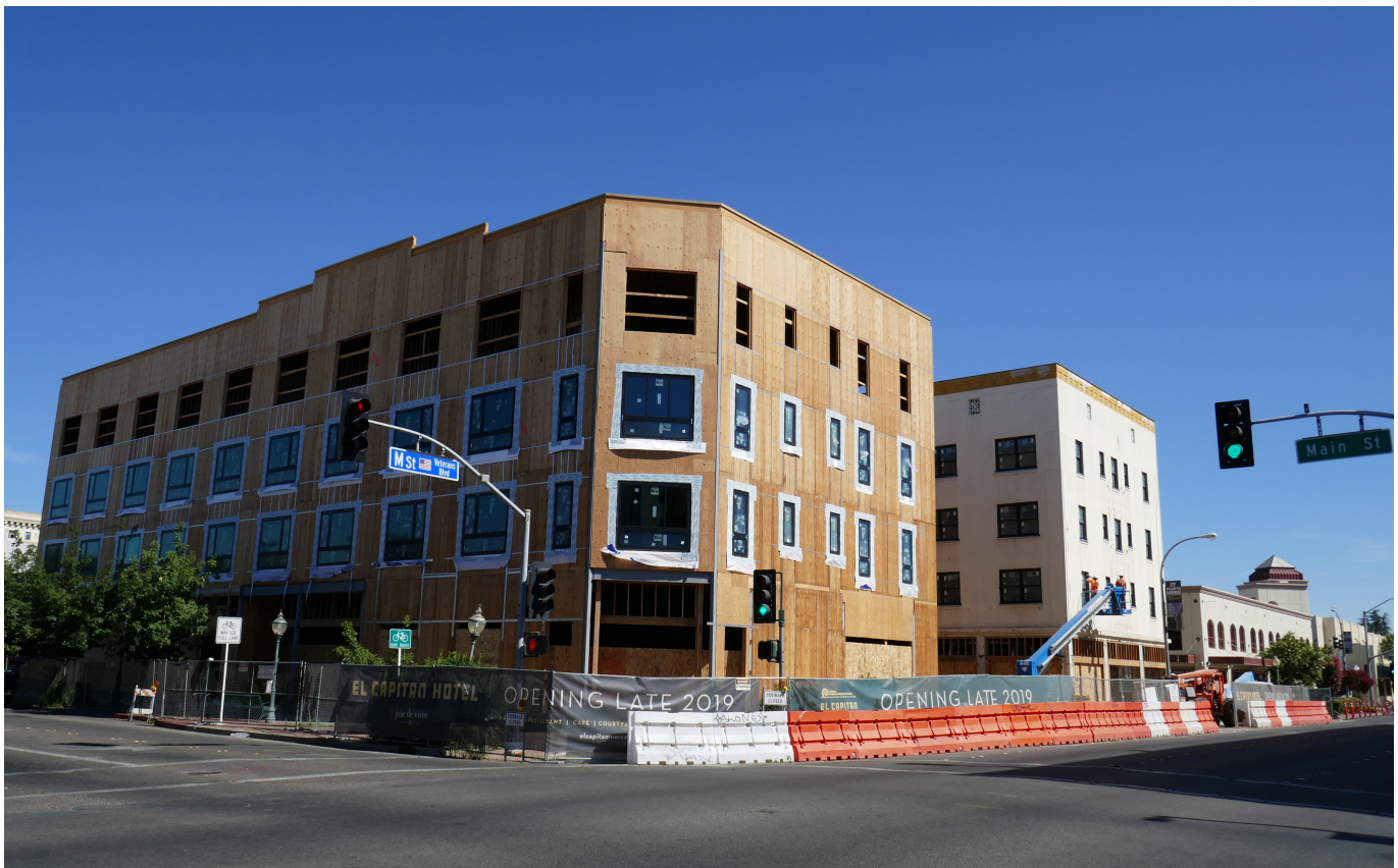
CIPAF 030 El Capitan Hotel Under Construction - Downtown Merced
