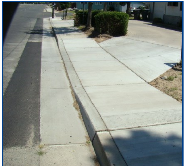
Work along Juniper Ave
