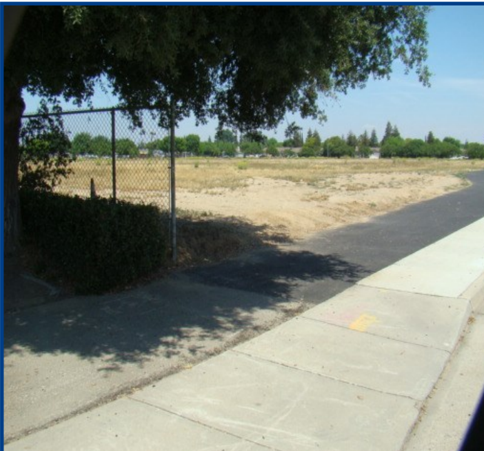
Work along Juniper Ave near Joan Faul Park
