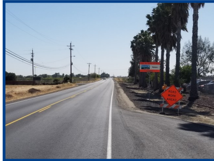
First Regional Project - Henry Miller Avenue Rehabilitation
