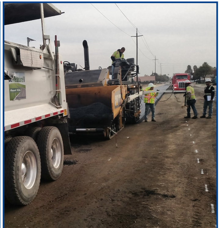
Pavement treatment on San Luis Street
