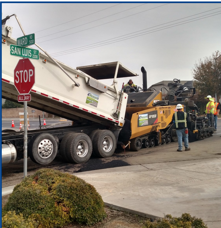
Pavement Treatment on San Luis Street and Ward Road
